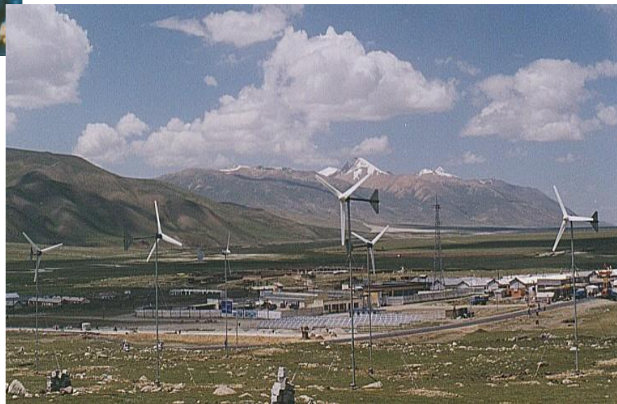
Wind/PV hybrid power station 风光互补发电站
